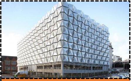
Building 106: Multi-storey car park
